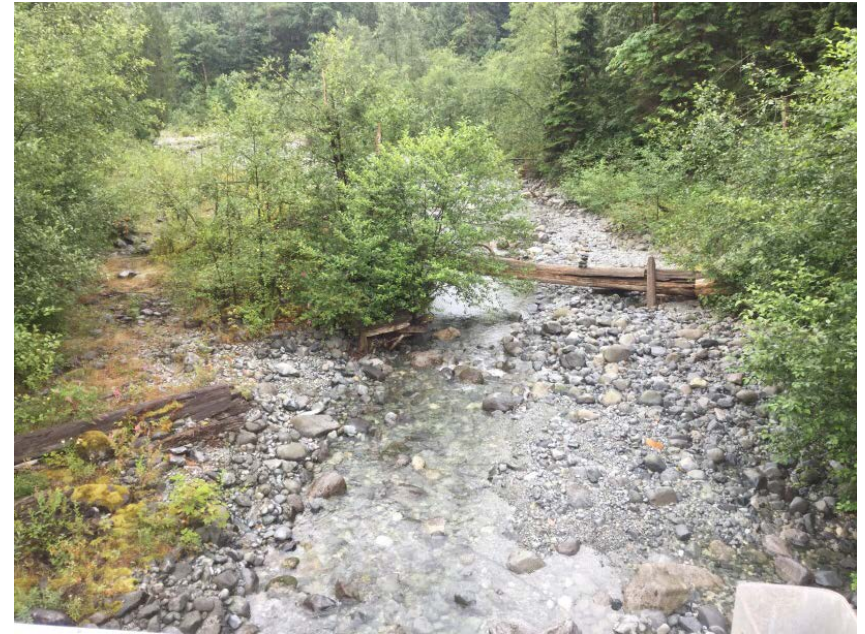
Looking downstream from deck
