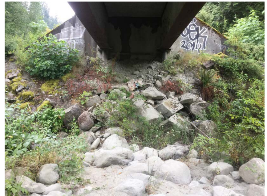
Left Bank Abutment when facing downstream
