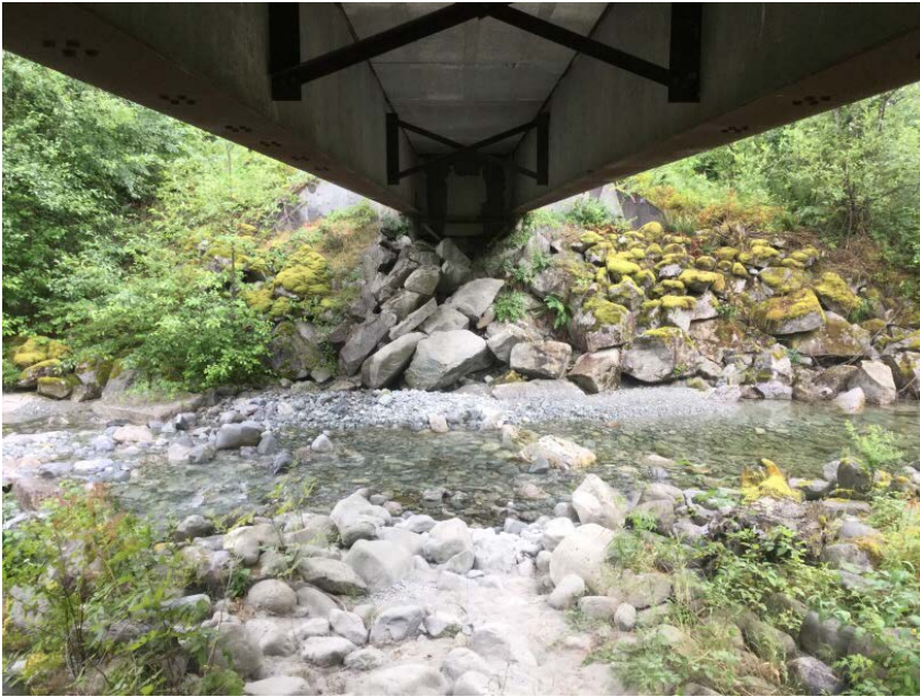
Right Bank Abutment when facing downstream
